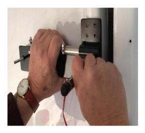
Offer back the deadbolt and insert the 5mm pop rivets and secure in place using pop rivet gun "not supplied".
