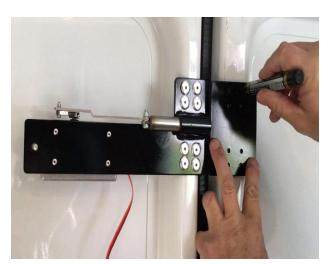
11/ On the side door offer up the deadbolt clasp make sure that the deadbolt will not hit the clasp; the bolt should slide through and not touch the clasp.
